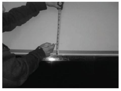
d) Level and screw the cleat to wall at the 3  $\frac{1}{4}$ " mark using the provided screws
